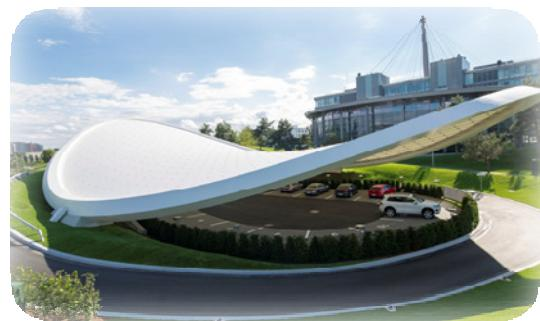
The surface of the roof is formed by extending the hyperbolic paraboloid surface **ABCD**.
