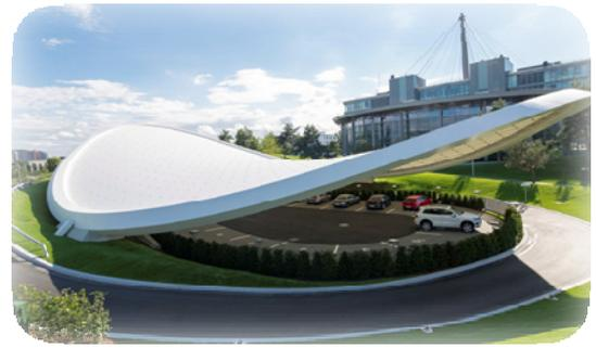
The projections of the roof are shown in Fig. C-2 below. The perimeter is an ellipse in plan. The lengths of the major and minor axes are 42m and 22m respectively.
