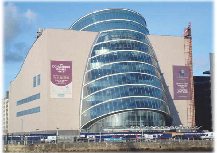
Fig. B-1 shows the elevation and end view of part of the structure. It consists of a portion of a right cylinder with its axis inclined at  $60^\circ$  to the horizontal plane, as shown in the end view. The cylinder intersects the vertical front face of the building, producing elliptical curves as shown in the elevation.
